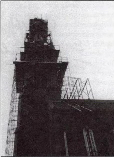
Three views of the steeple as it is dismantled. The scaffolding alone cost $90,000 to erect. Facing page: The steeple as it appears today.
