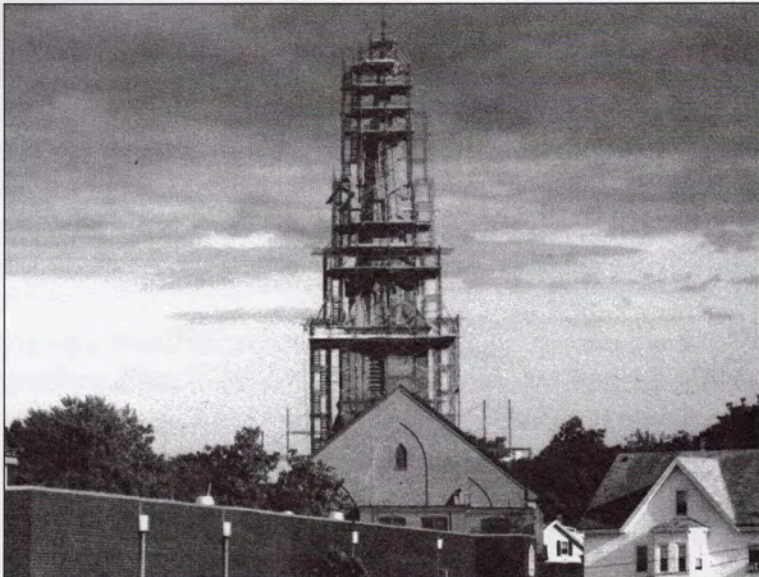
Three views of the steeple as it is dismantled. The scaffolding alone cost $90,000 to erect. Facing page: The steeple as it appears today.
